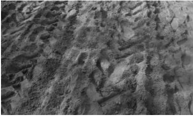
(a) Compacted soil used as sub-grade
